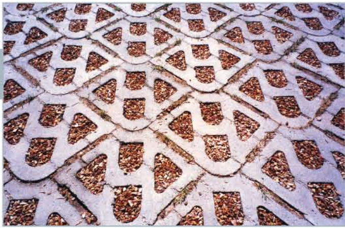
CANAL LINING/FLAT ROOF INSULATION
