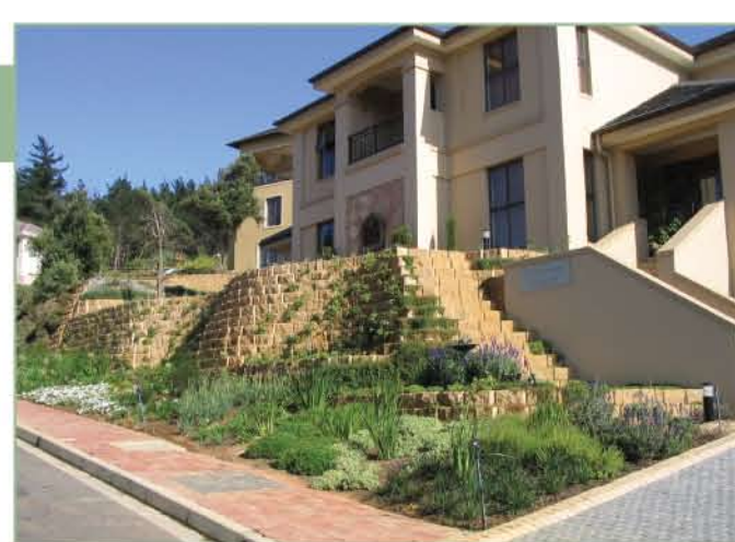
STABILISING AND LANDSCAPING OF CUT AND FILL SLOPES
